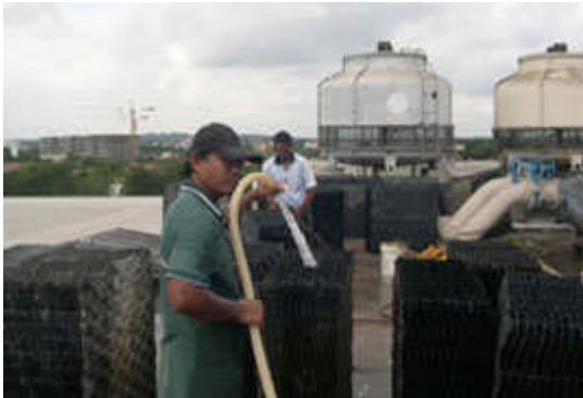
Descaling of Cooling Tower
