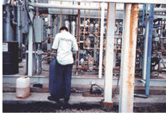
Descaling of Heat Exchangers
