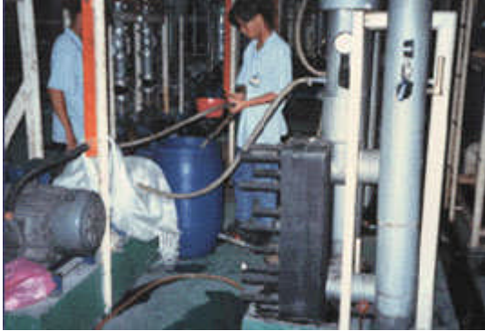
Descaling of machinery cooling channels
